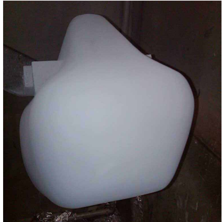
Maxium BHT-L applied by brush before drying
